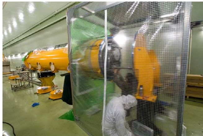
Beam pipe connection
