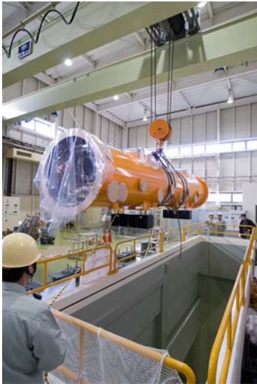
carrying down the cryomodule
