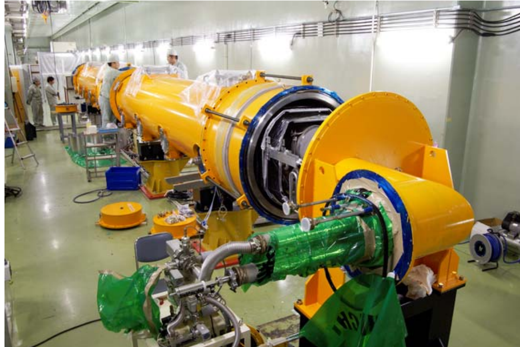
cryomodule sit in the tunnel
