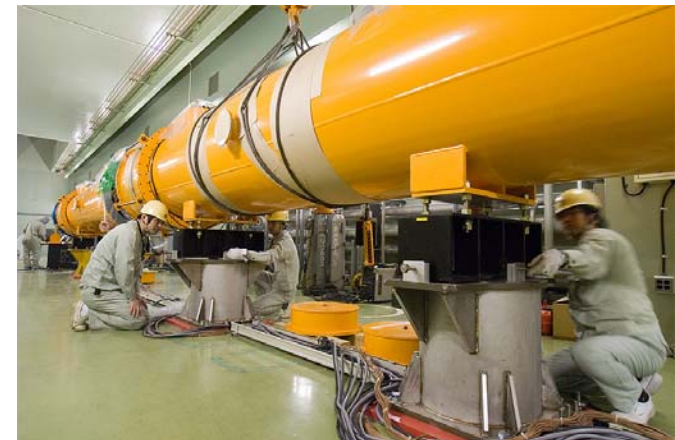
Downstream module installation
