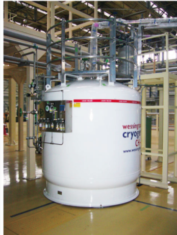
3000L liquefied helium storage vessel
