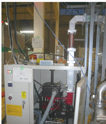
30kW CW IOT for main SCC
