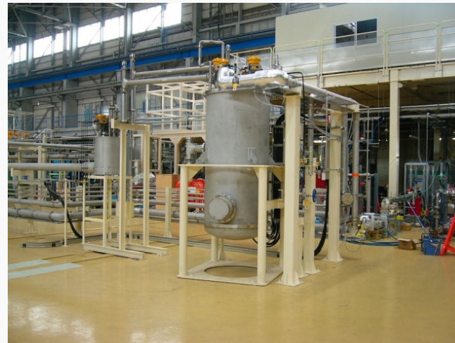
2K cold box and end box
