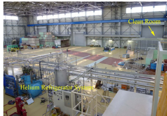
Figure 4: East Counter Hall after the refurbishment.
