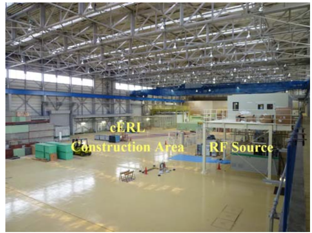
Figure 6: The inside of the East Counter Hall after its refurbishment.
