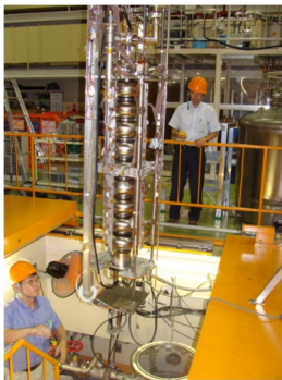
Figure 4 : Installing 9-cell cavity to cryostat
