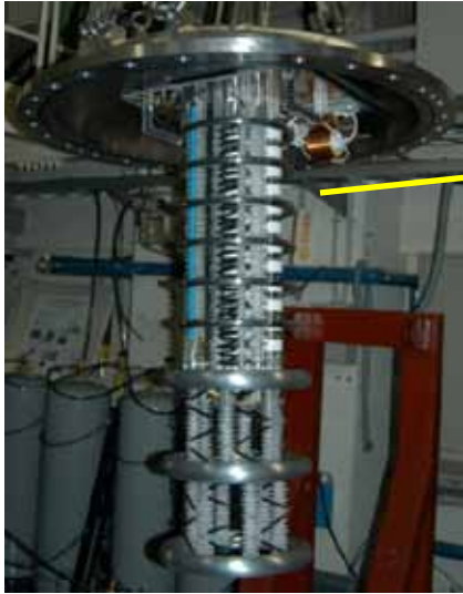
550kV Cockcroft Walton power supply
