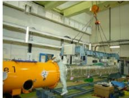
Insertion into vac. vessel 1 week
