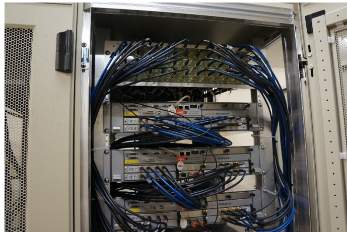
Figure 5: A part of the new beam position circuits installed into the standard rack.
