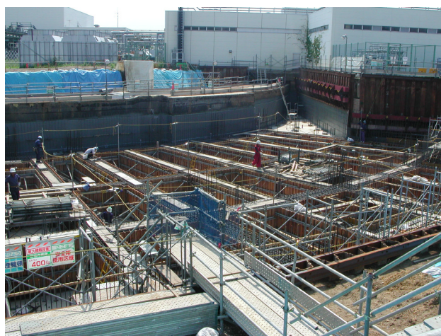
Figure 6. NW experimental hall is now under construction.
