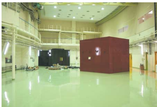
Figure 5 AR-NW12 beamline under construction. The black box in the back is an optical hutch, which contains optical elements such as collimating mirror, cryogenically cooled double crystal monochromator and a focusing mirror. The brown box in front is an experimental hutch, in which an X-ray camera specialized for MAD measurements of protein crystals will be installed.
