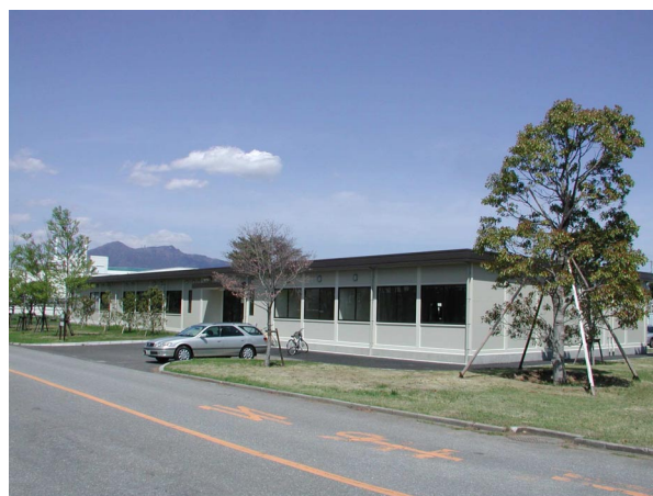
Figure 2 The Structural Biology Building after the extension in March 2003.
