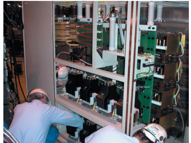
Figure 18 Installing the high-voltage cabinet for the new klystron power supply.
