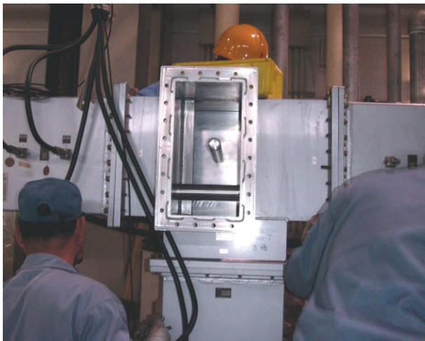
Figure 3 Installation of an asymmetric power divider into the PF-AR system.
