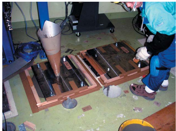
Figure 13 The base plate of the magnet girder.
