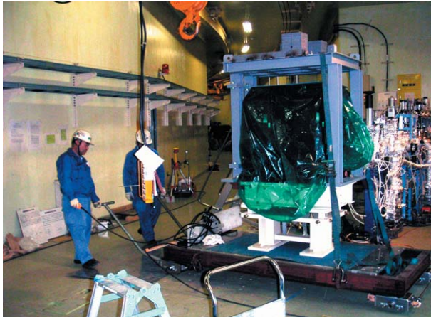
Figure 14 Installation of a new quadrupole magnet.
