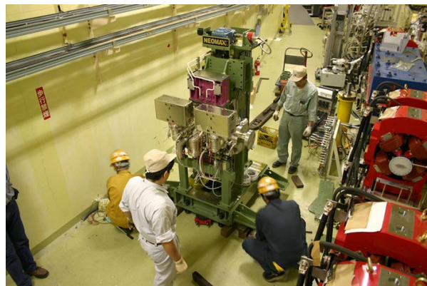
Figure 8 Installation of SGU#17.
