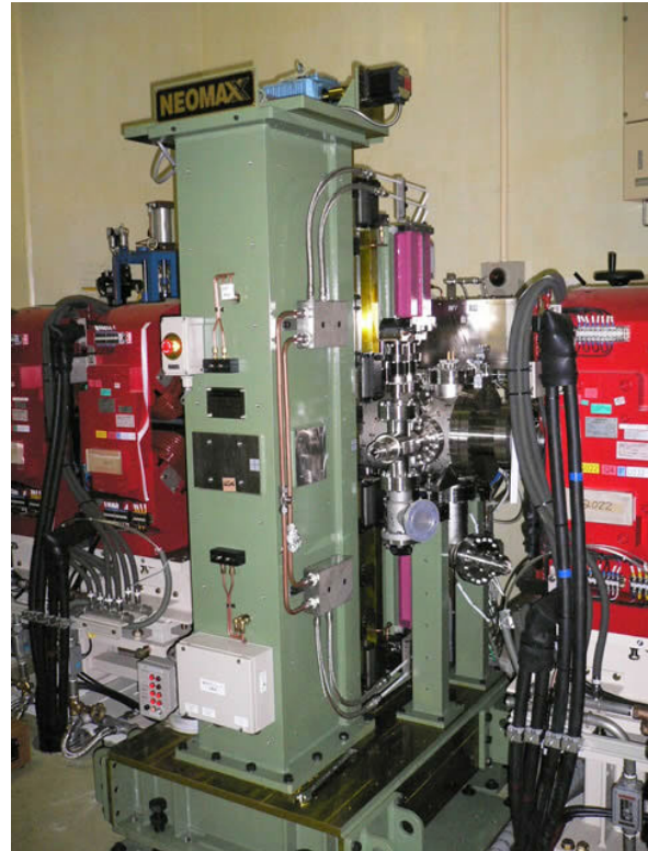
Figure 21 Installation of SGU#03.
