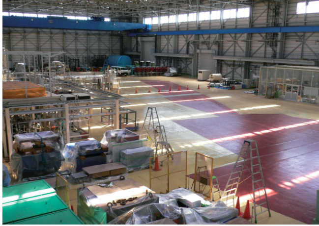
Figure 7 View of the ERL Test Facility after its renovation and clearing.
