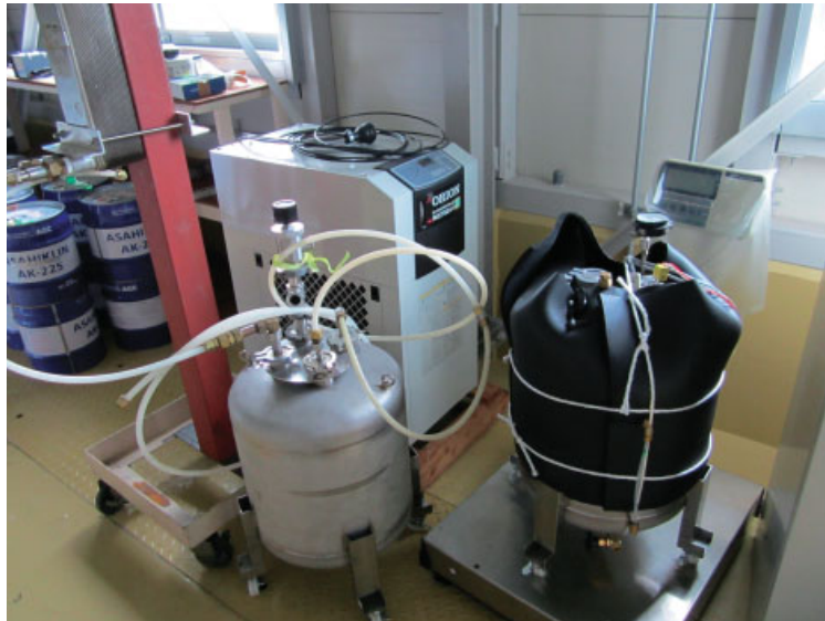
Figure 32 Hand-made distiller unit (two storage vessels and one heat exchanger on a red post) for purifying oil solvent from tubing inside the helium liquefier/refrigerator.
