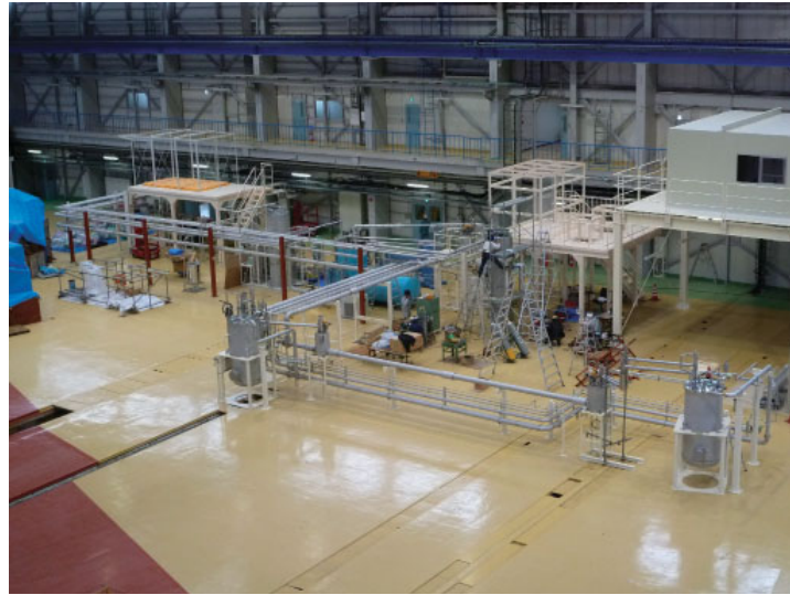
Figure 29 2-K helium cryogenic system for cERL; Two 2-K helium refrigerator cold boxes are ready to be connected to cryomodules of superconducting RF cavities for the injector and main linacs.
