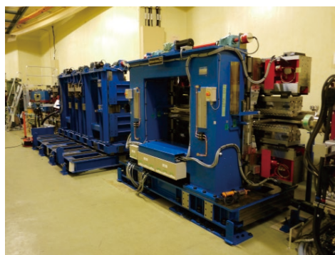
Figure 7: U#02-1 and U#02-2 during installation.
