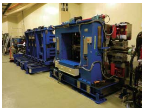
Figure 7: U#02-1 and U#02-2 during installation.
