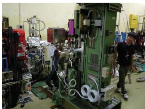
Figure 5: SGU#15 during installation.
