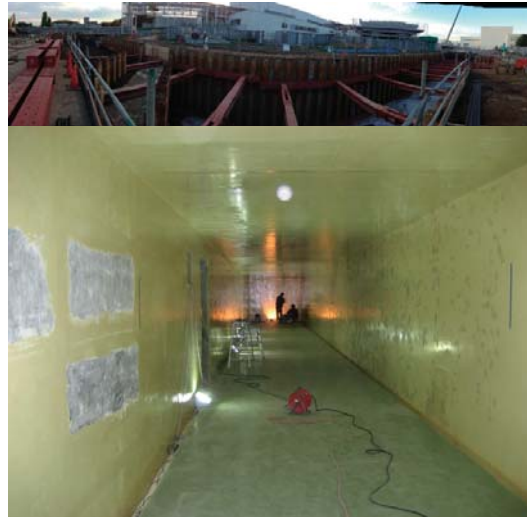
Figure 4: Upper photograph: the precursor tunnel in November 2013. Lower photograph: the inside of the tunnel before painting.
