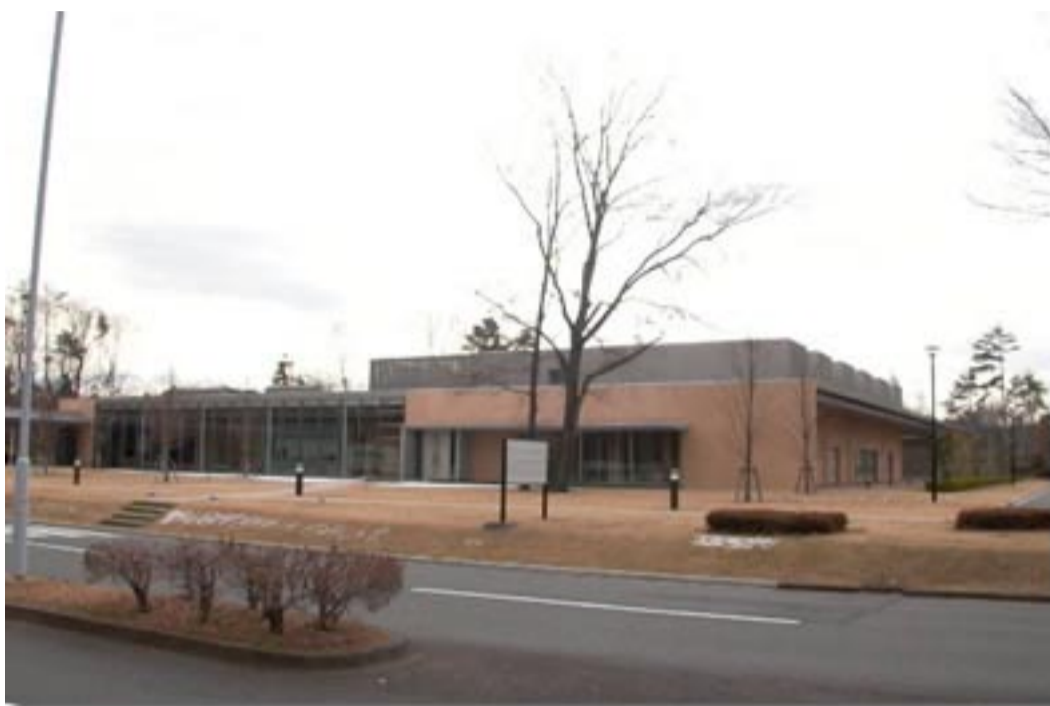
Conference site: Lounge 1&2 in KEK International Center
