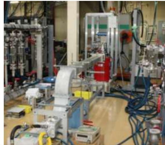
30kW CW Klystron for injector SCC
