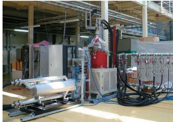
Figure 17 300-kW klystron system installed in the ERL Test Facility.
