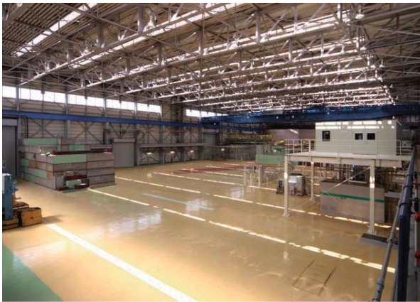
Figure 6 View of the ERL Test Facility after renovation.
