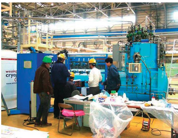
Figure 19 Helium liquefier/refrigerator that is installed in ERL Test Facility.
